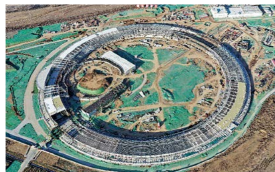
An aerial view of HEPS project site (photo in Dec. 2020)
