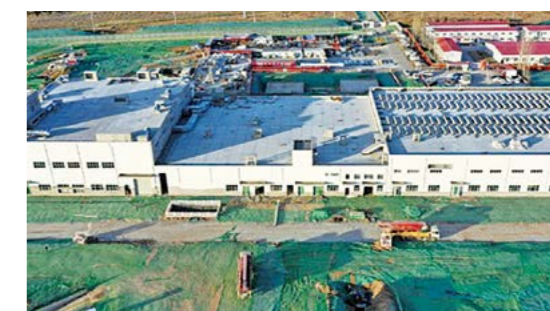
Roof-sealing work for the utility building was conducted on May 18, 2020.
