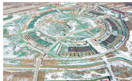
An aerial view of HEPS project site (photo in Jan. 2020)
